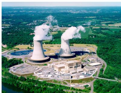
The Limerick Station: Twin General Electric 1143MW boiling water reactors punctuated by twin 507 ft. natural draft hyperbolic cooling towers. Shantego, Pennsylvania.
